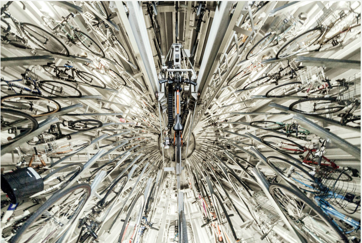
Figure 37: Smart multi-level underground bike parking in Tokyo, Japan
